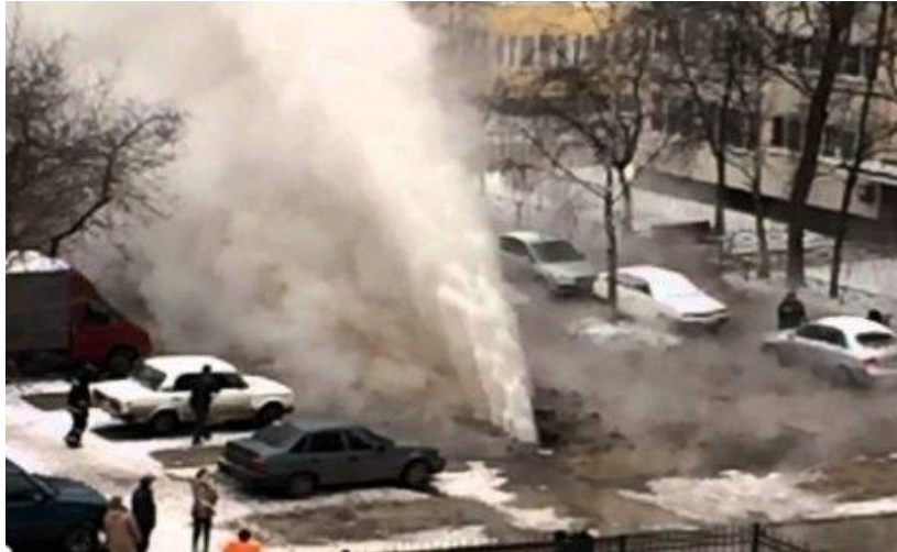
Figure 2. Pipeline explosion in Almaty city
